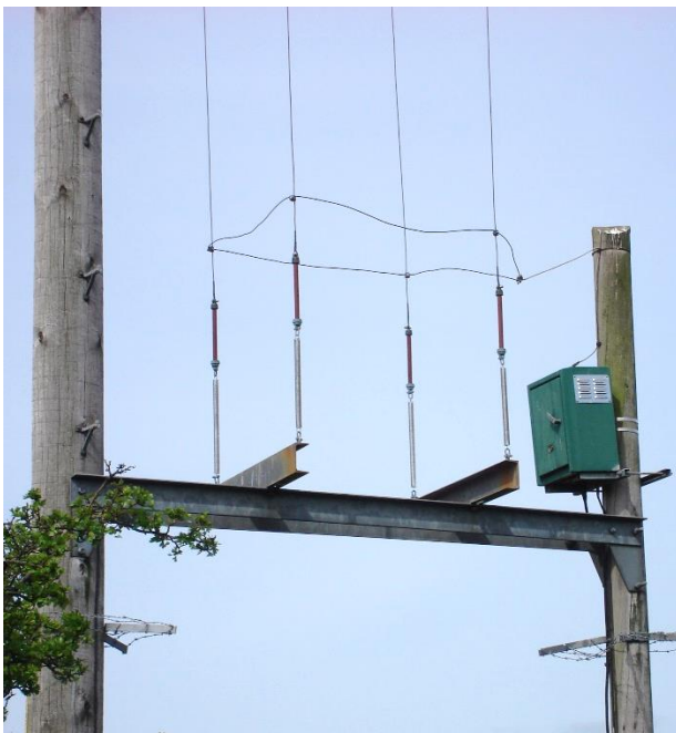
Figure 8. Worcester MF antenna termination. Photo: Ian Chalmers G8HON
